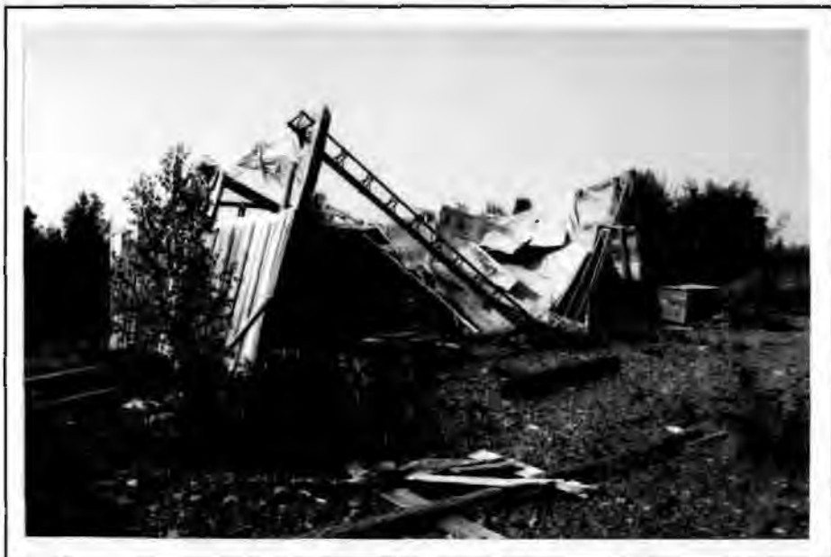
Figure 104. The Fullerton Hanger, 1993. The view is looking southwest.
